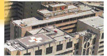
Grady Memorial Hospital Helipad Apr 19, 2012 | Hospital Heliports, Rooftop Heliports
