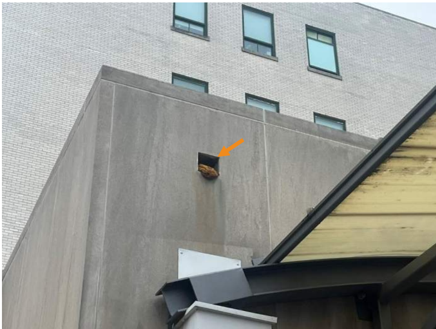
Figure 64. Openings in the limestone panel at the base of roof parapet walls.
