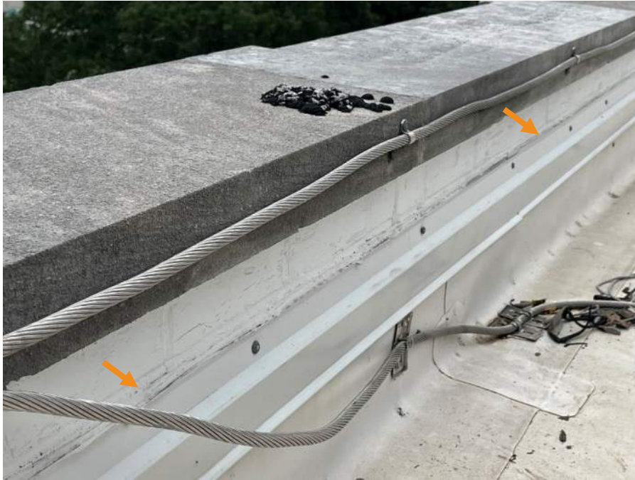
Figure 105. Roof membrane counter flashing termination at the interior face of the parapet with coated brick.
