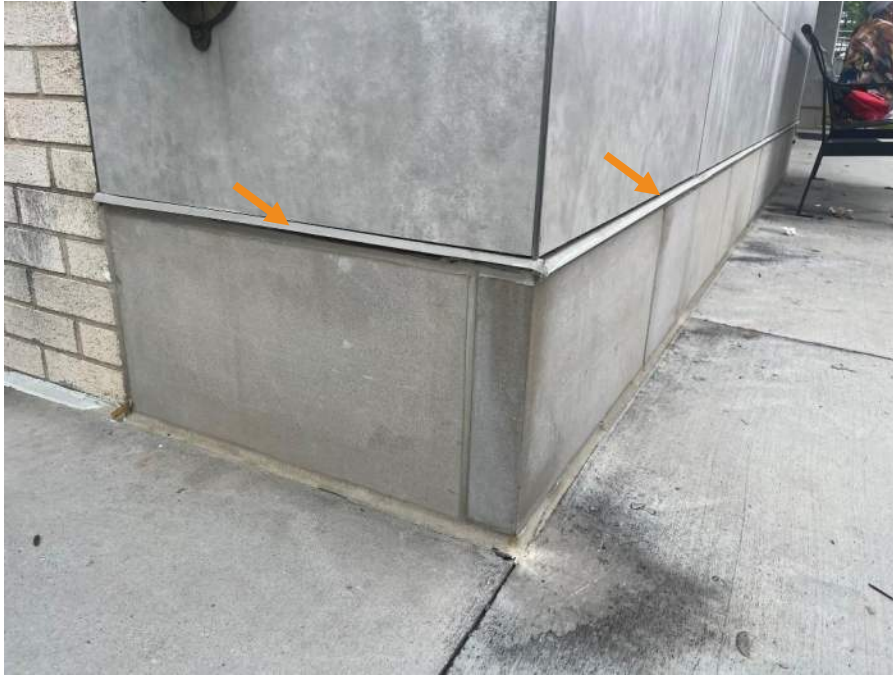
Figure 81. Flashing daylighted one course above grade.
