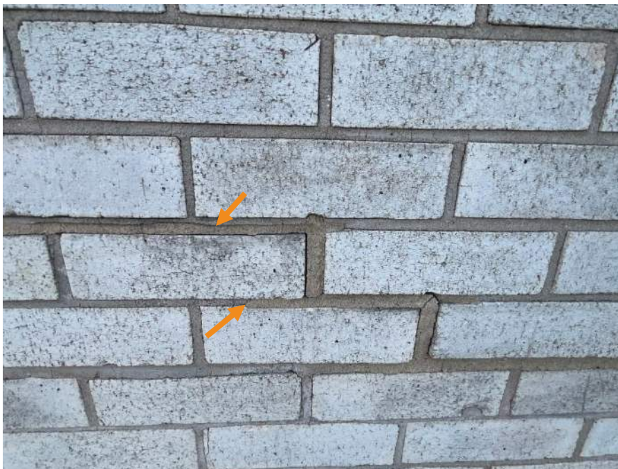
Figure 26. Location of varying mortar finishes and colors.
