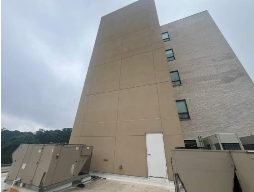
Figure 69. Overview of EIFS at west elevator tower
