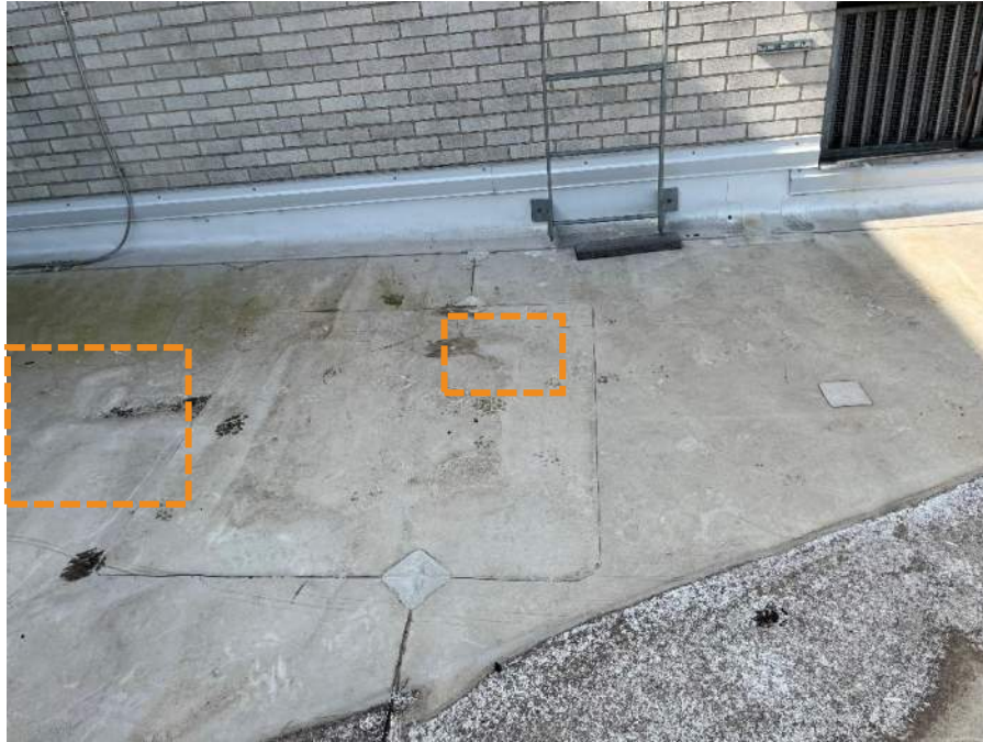
Figure 103. Isolated blisters at crickets
