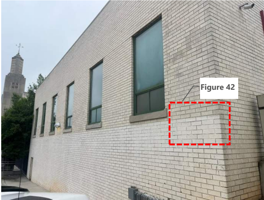
Figure 41. Coating applied to brick face from Level 2 floor line and below.
