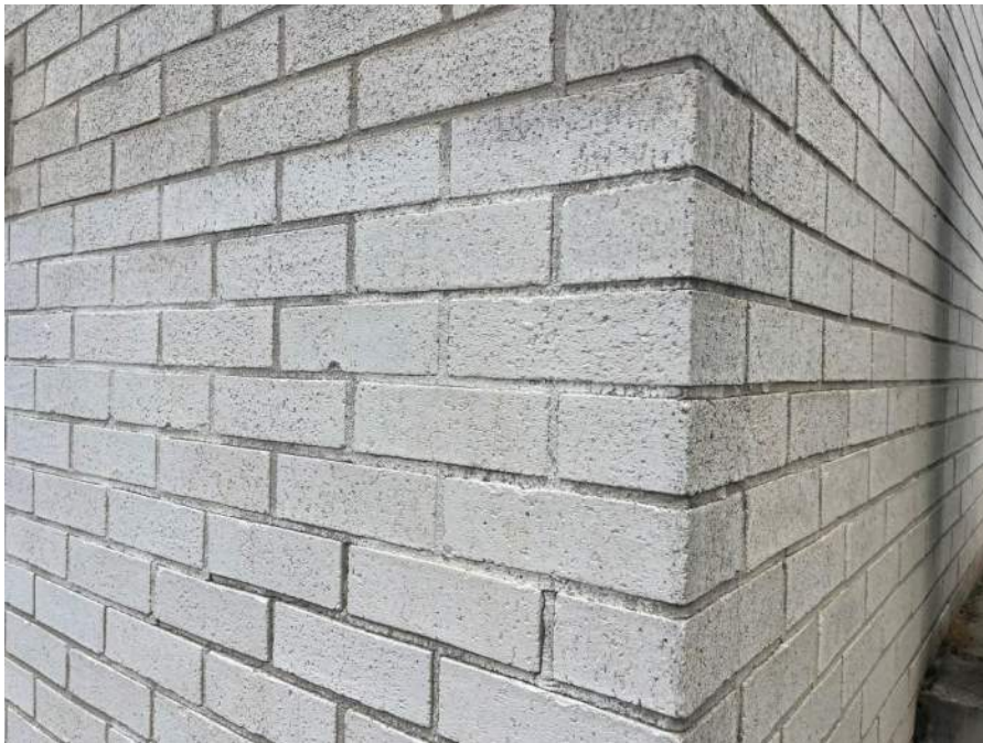
Figure 42. Close-up view of white coating applied to east wing south facade
