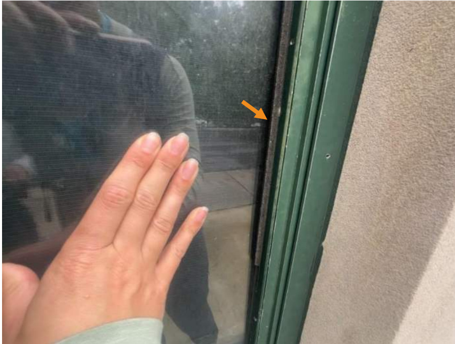
Figure 93. Acrylic panel at north facade ground floor window unit able to be displaced inward
