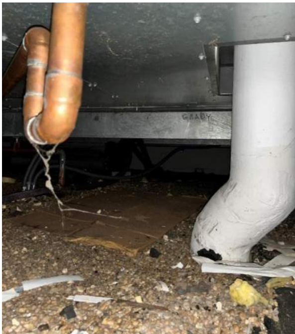
Figure 112. View from interstitial space between the mechanical system and roof below, exposing built-up roofing assembly and pipe penetrations below
