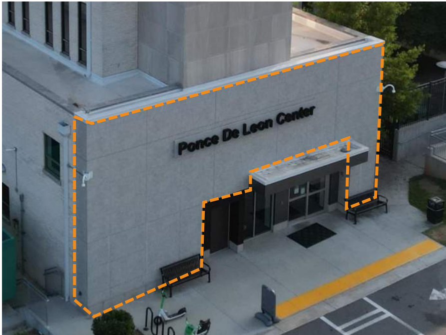
Figure 77. Porcelain tiles installed at main building entrance
