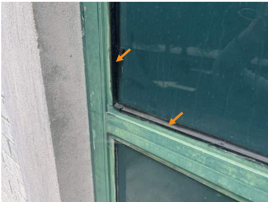
Figure 92. Sealant installed at glazing-to-metal transitions at north facade window
