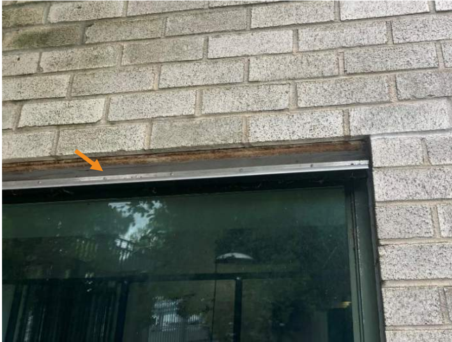
Figure 85. Gray sealant installed along the leading edge of the face fastened drip edge.
