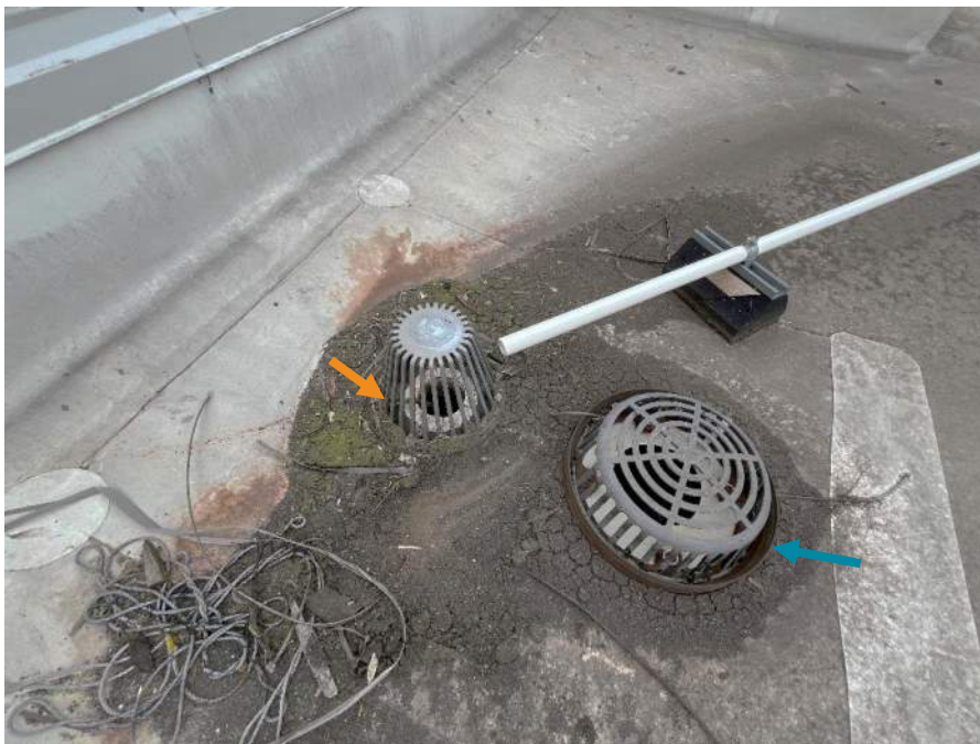
Figure 94. Primary drain (orange arrow) and overflow drain (blue arrow) at main roof
