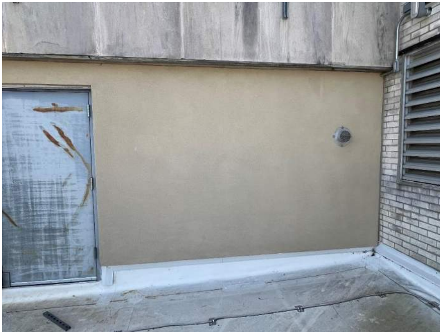
Figure 70. Overview of EIFS at mechanical penthouse west facade
