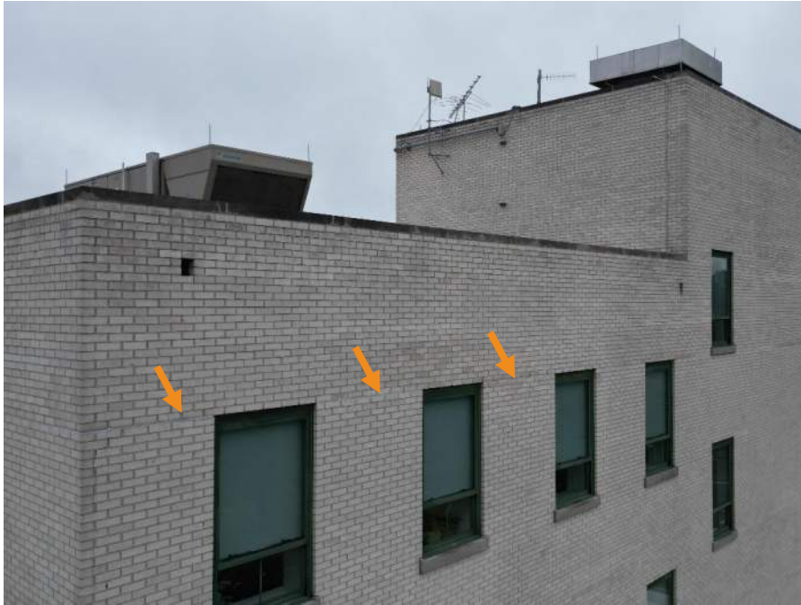
Figure 33. Sealant installed at bed joints aligned with window heads.
