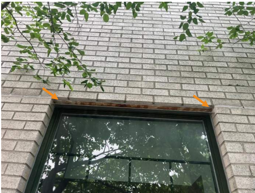
Figure 86. Sealant applied along the exposed lintel at a window on the courtyard west facade.
