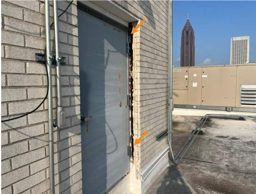
Figure 21. Stairwell access door to main roof set back from brick masonry face.
