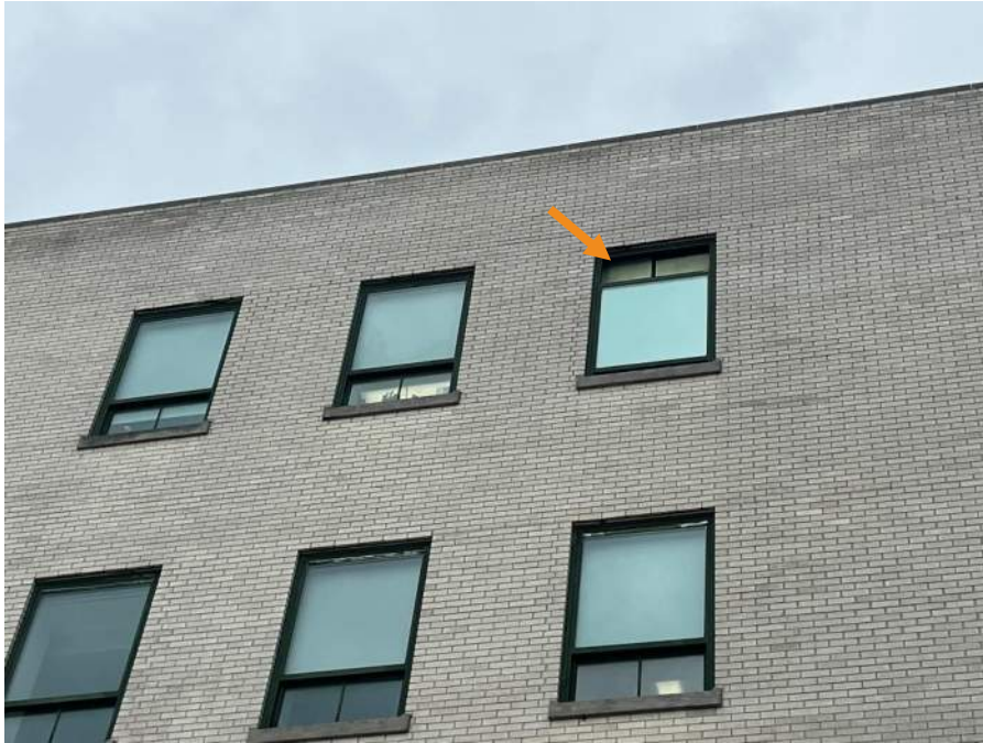
Figure 89. Open window at the east facade.
