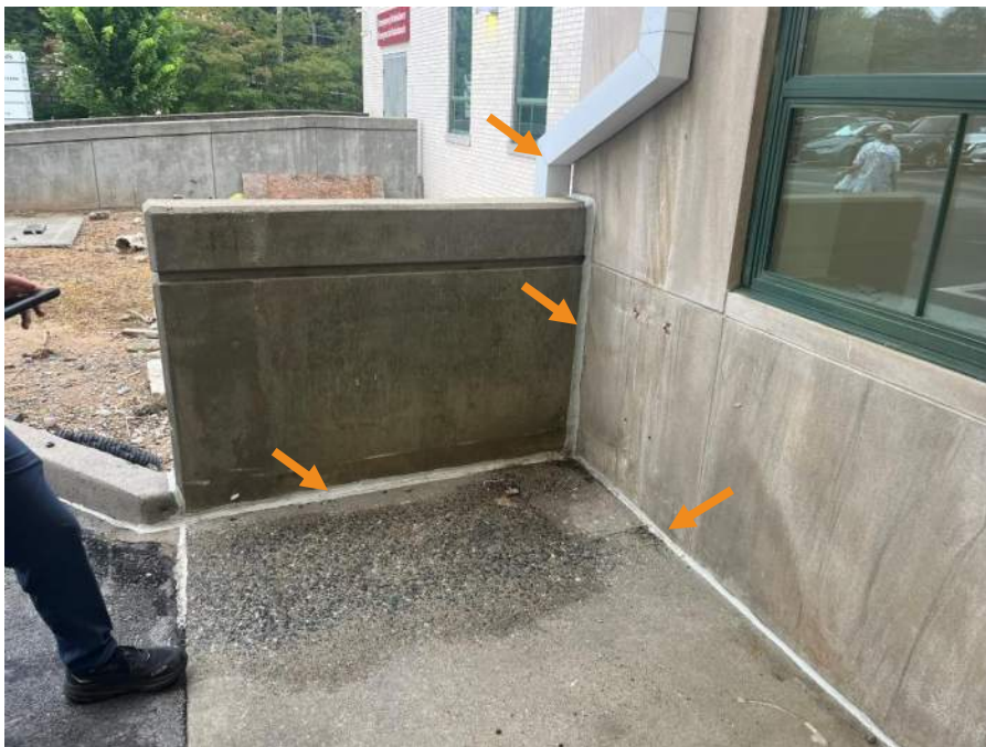
Figure 62. Downspout and sealant installation adjacent to the east facade employee entrance.
