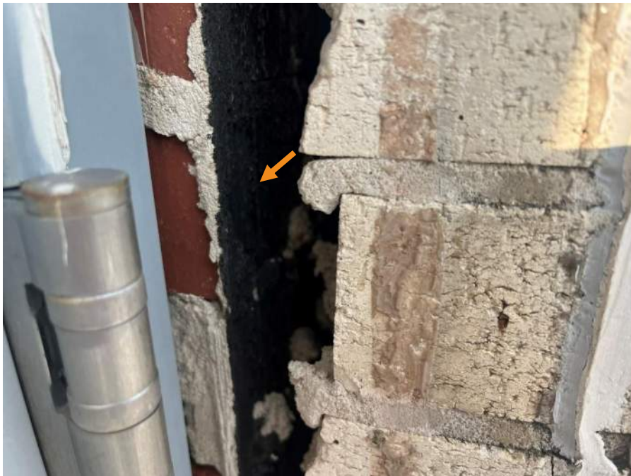
Figure 22. Exposed two-inch drainage cavity and dampproofing (orange arrow) applied to brick masonry backup wall.
