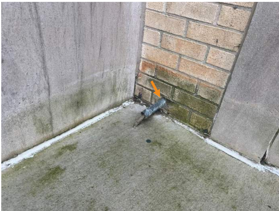
Figure 40. Mechanical penetration on the north facade at grade.
