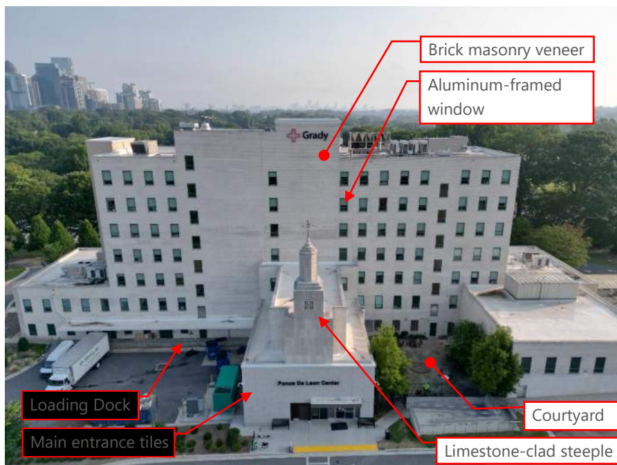
Figure 2. Aerial view of the Ponce De Leon Center south facade
