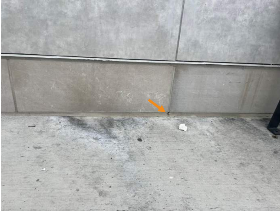
Figure 61. Sealant with exposed tube weeps installed between the limestone panels and concrete sidewalk at grade.
