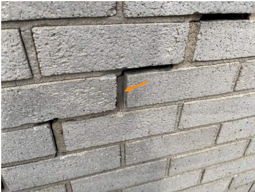
Figure 30. Saw cuts creating crescent profile in head joint.
