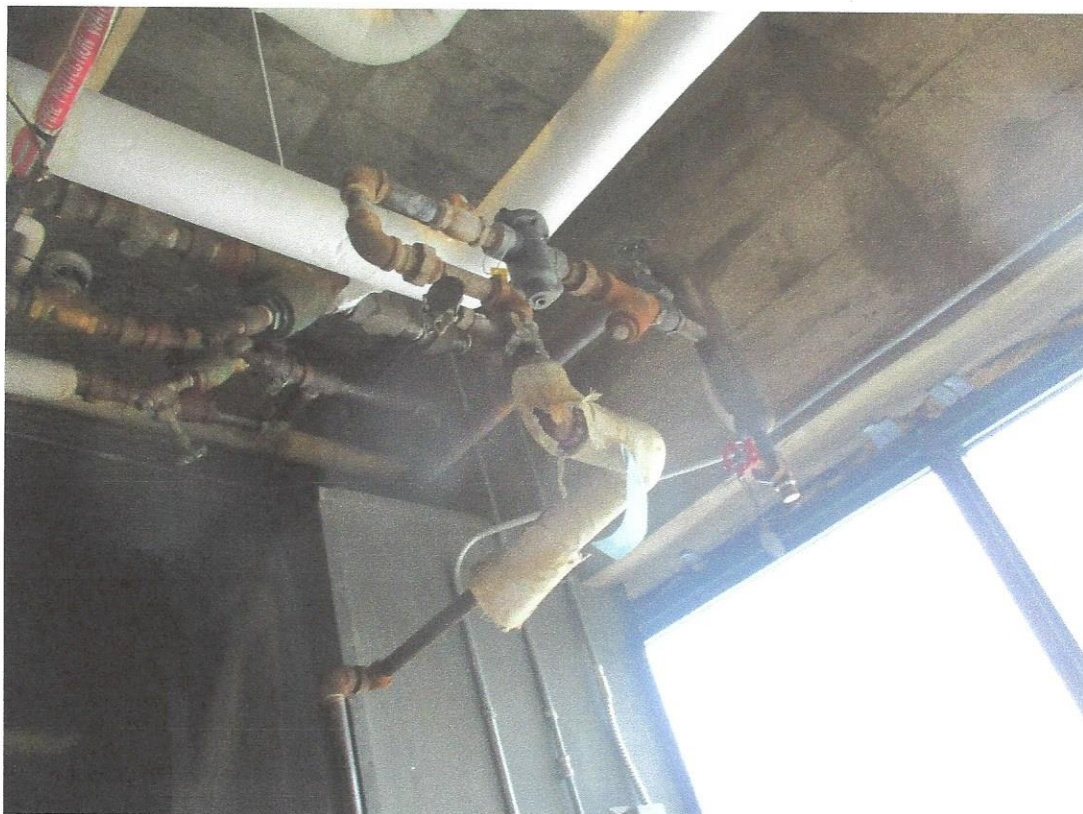
Photo #6 – TSI, piping and pipe fittings, cementitious - PACM*
