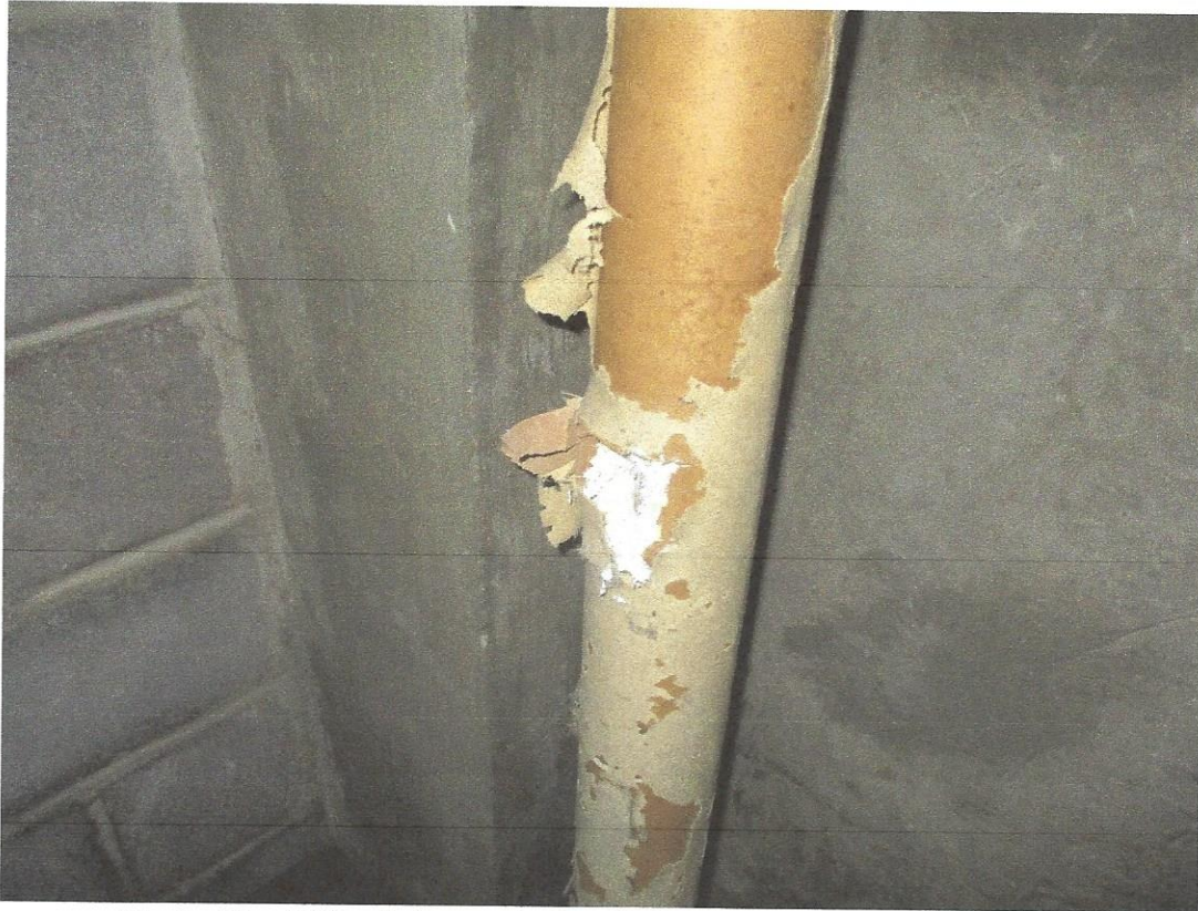
Photo #7 – TSI, piping and pipe fittings, cementitious - PACM*
