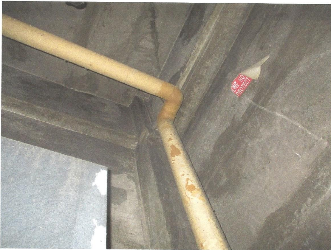
Photo #8 – TSI, piping and pipe fittings, cementitious - PACM*
