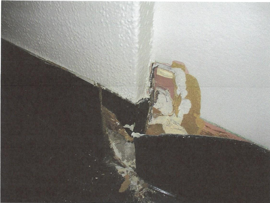
Photo #4 – Wallboard with red backing and joint compound
