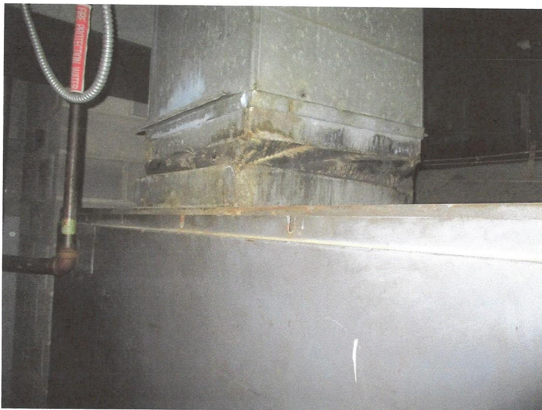
Photo #10 – Vibration dampeners - PACM*
