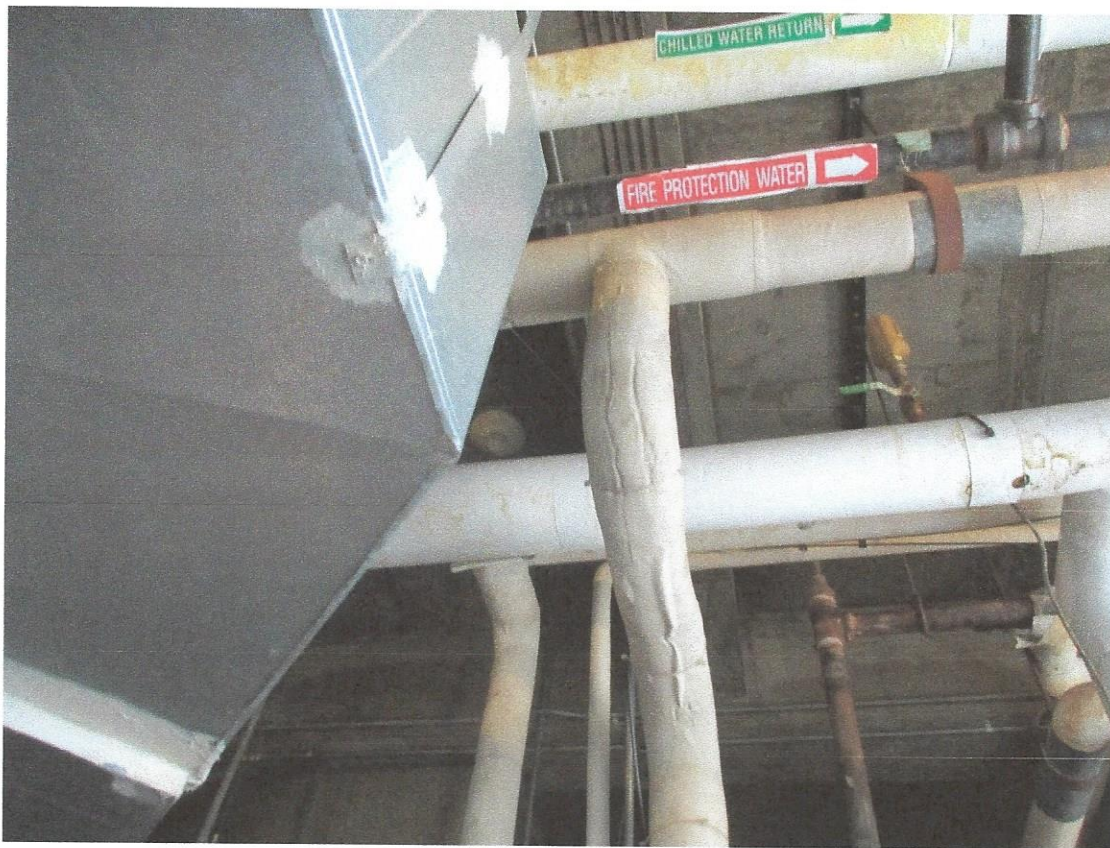
Photo #5 – TSI, piping and pipe fittings, cementitious - PACM*
